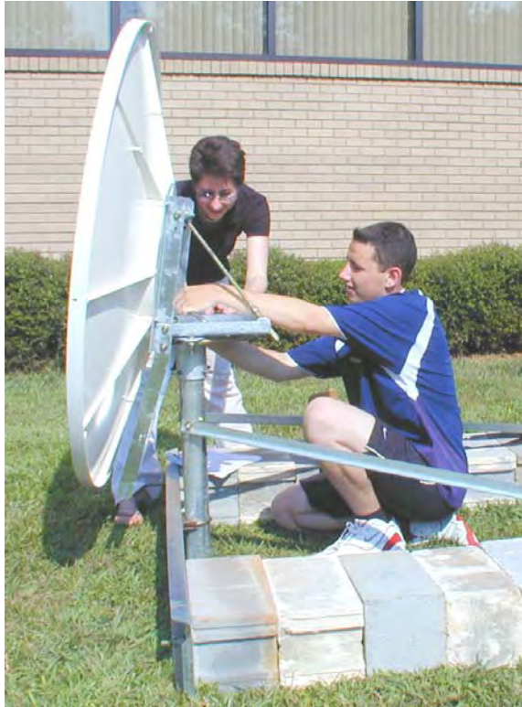
Fitting the reflector to the mount.
