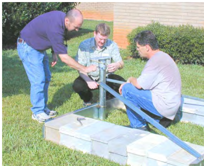
Assembling a non-penetrating mount for a 1.2 meter antenna.
